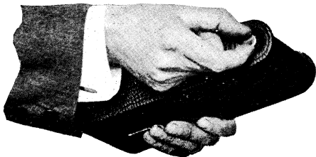
FIG. II. Springing Out a Spool Pin.
